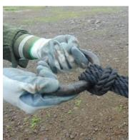
Once knotted through the steel ring, the FRN Gabion is safe to be lifted using the same ring. The filled FRN Gabions can be directly installed using lifting equipment or transported and installed in required sites. Ensure safe working conditions at all times.
