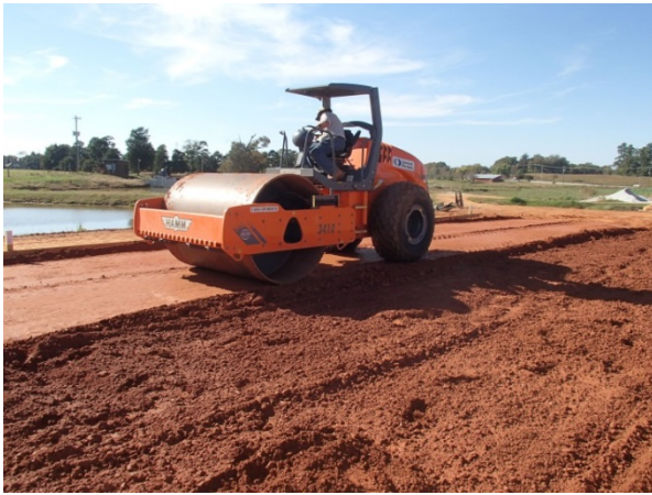
Figure 2: Sub-Base Compaction
