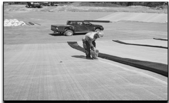
Seaming Bentonite Granules placed on Bentoliner EB (a) using dispenser or (b) using plastic watering bucket
