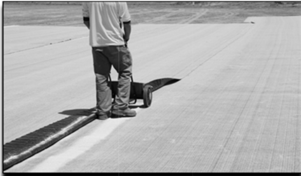
Seaming Bentonite Granules placed on Bentoliner EB (a) using dispenser or (b) using plastic watering bucket
