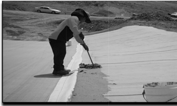
Seaming Bentonite Paste used on transverse joins
