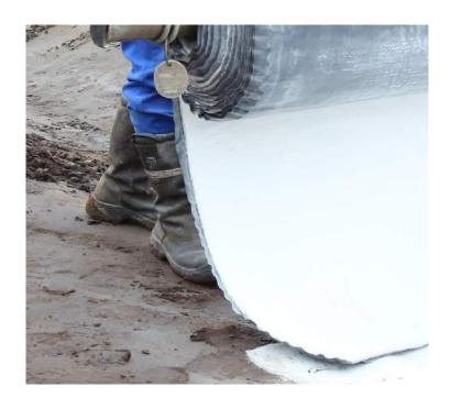
For easier handling and positioning it is recommended to provide a lifting device which allows to lift the rolls with a front end loader. The iron core may serve as a device for unloading as well as for installation of the liner. The orientation of panels on slopes shall be parallel to the slope. The panels should be anchored to the trench at the top of the slope. When setting subsequent layers ensure there is at least a 10 cm overlap between layers in the direction of water flow.
