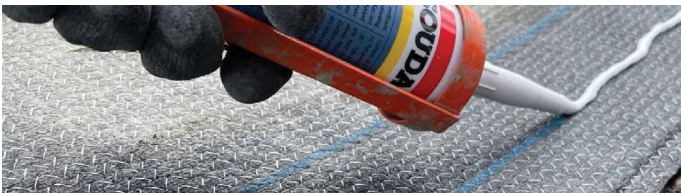
Figure 9. Sealant applied along fixing marker line
