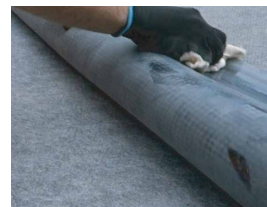
Wipe clean the LLDPE backing
