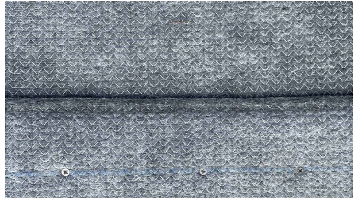
Figure 7. Screws inserted through fixing marker line
